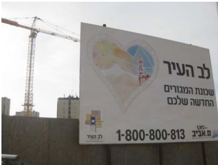
Fig. 3d: Lev ha-Ir neighborhood construction complex
